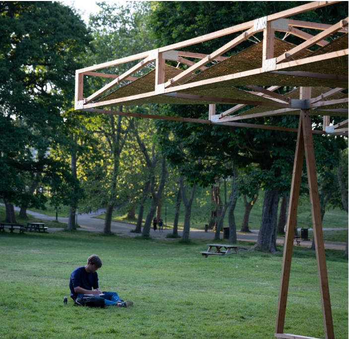
IMAGE: Architecture practice Studio Saar produced the Craft Not Carbon pavilion in London’s Crystal Palace Park for the 2023 London Festival of Architecture. The structure uses a woven bamboo canopy made by local craftspeople, that can be repaired by local weavers after storms.
